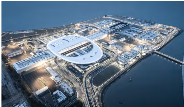
Hong Kong-Zhuhai-Macao Bridge
